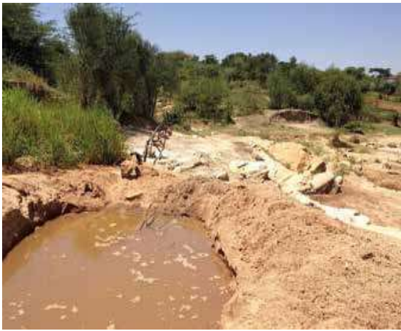
Fig.4. a sand storage dam connected to a small-Scale irrigation system in Kenya. Photo: J. de Trincheria.
