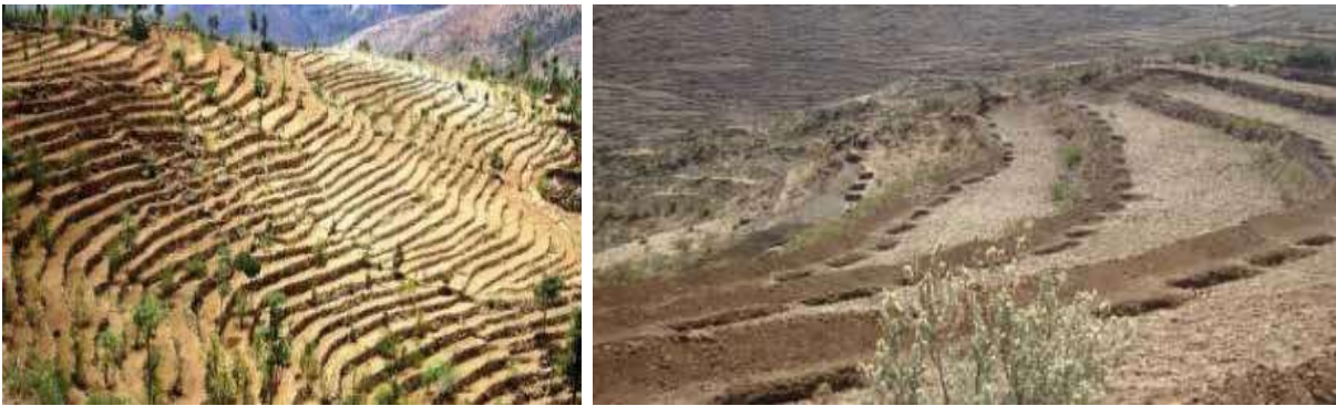
Figure 3: Micro-catchment RWH systems (terraces -left- and trenches -right-) that are infiltrating rainwater and higher shallow groundwater levels in Ethiopia. Photo. B. Simane.
